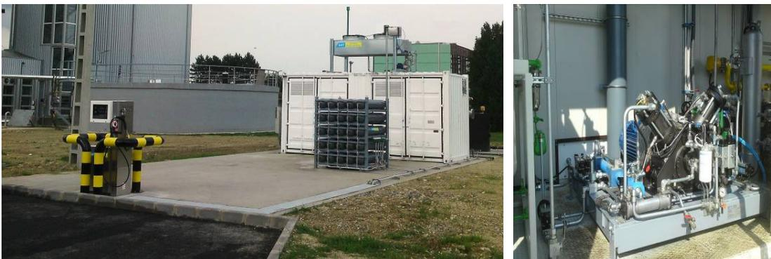
**Figure 12: Photo impression of small scale upgrading plant including compression to 220 BAR, STORAGE AND DISPENSER.**
